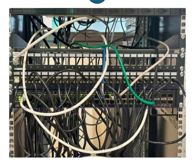
Ci-dessus un switch Cisco SG500X 48 ports 10 Giga SFP+.
